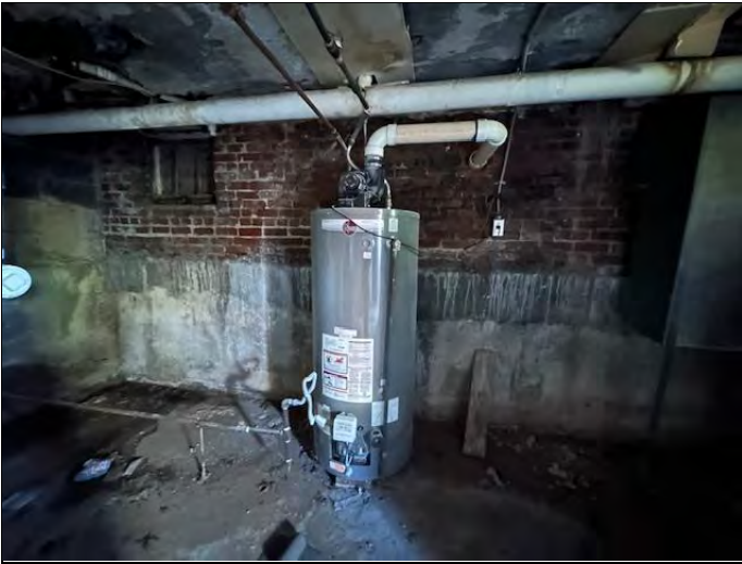
19. Gas-fired central water heater
