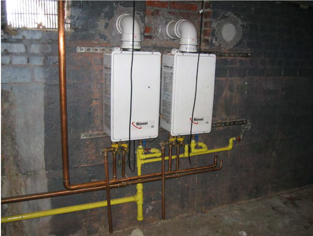
Newer tank less water heater system in Building 9
