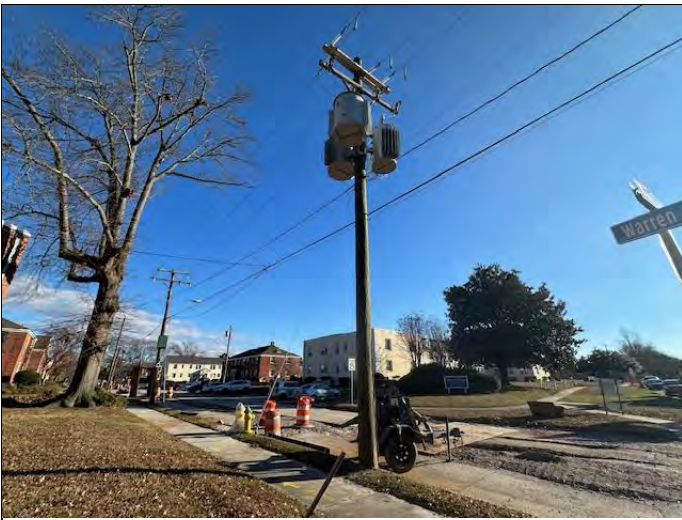
27. Pole-mounted electrical transformers
