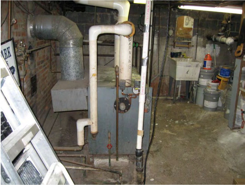
Common gas fired boiler system provides comfort heat in some buildings
