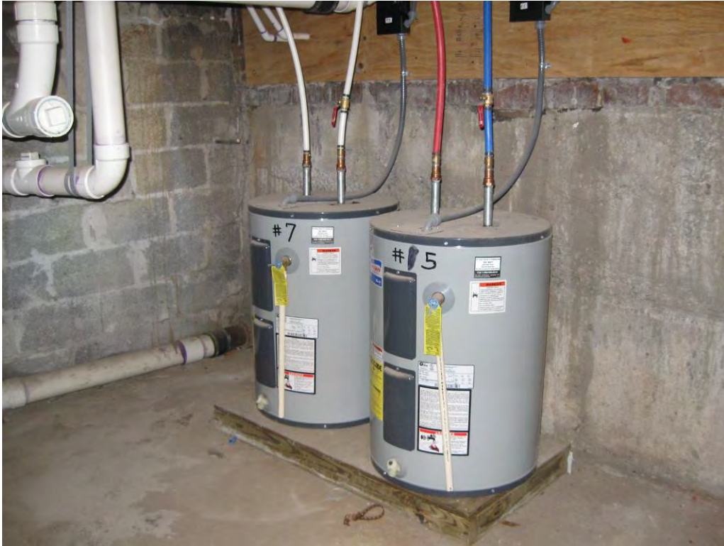
Building 19 have newer individual electric water heaters and newer PEX water supply line piping
