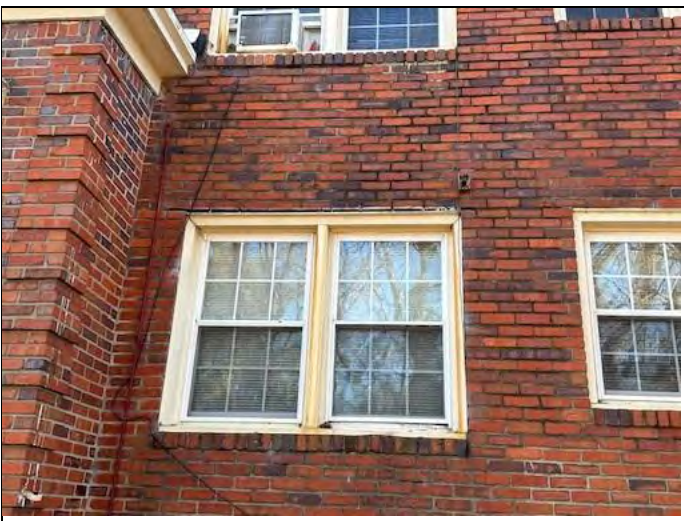
59. Representative cracking and separation at façade (Bldg. 8)
