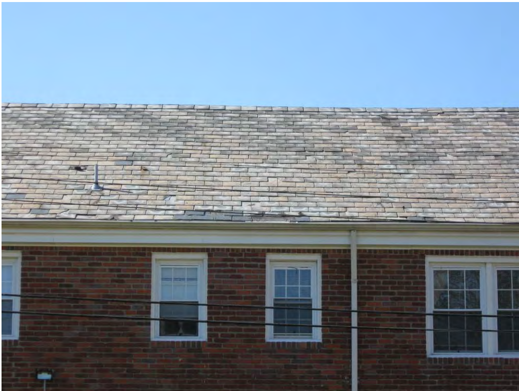
Slate roofing shingle maintenance required on some buildings (Bldg. 22)
