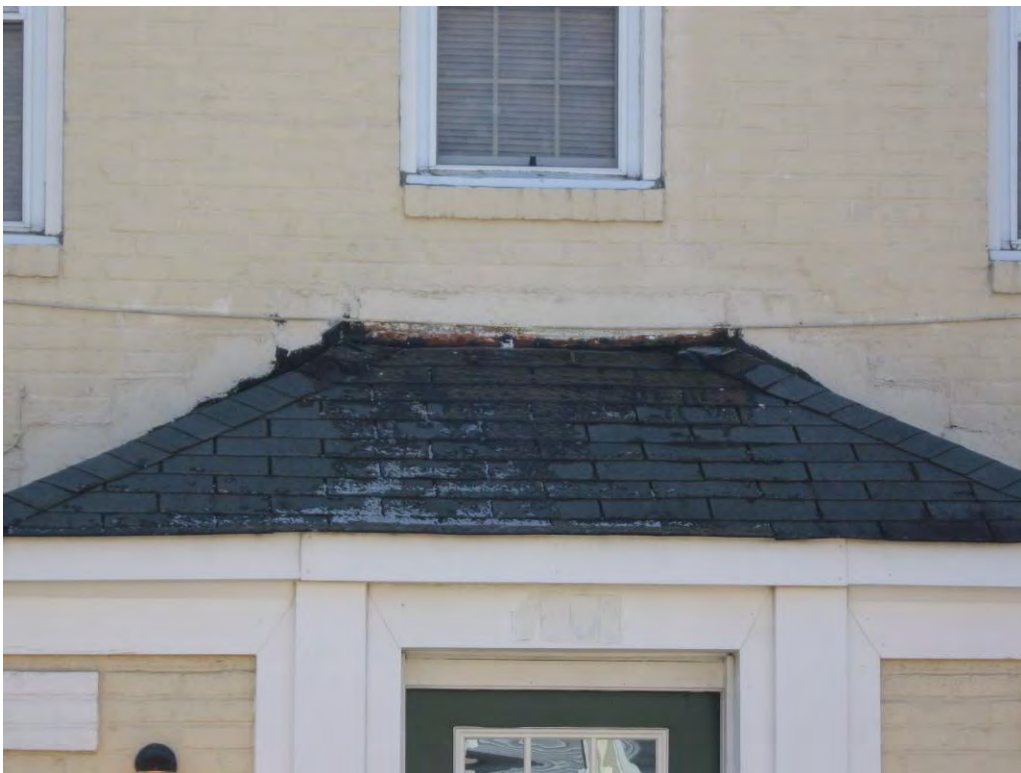
Roof flashing repair required (Bldg. 5)
