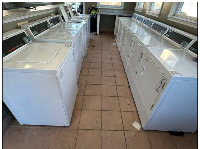
36. Laundry facility top load washer and front load dryers; note lack of sufficient clear space
