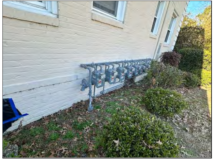
26. Natural gas regulators and meters
