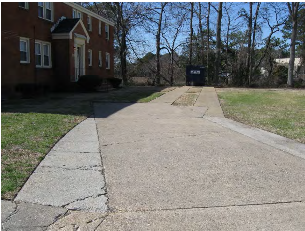
Concrete service drives located throughout site, concrete flatwork repairs required in several locations
