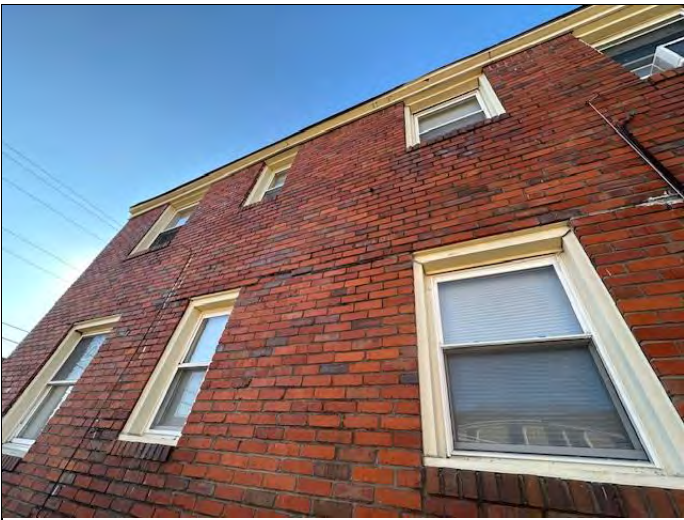
57. Representative exterior façade cracking and gapping above ground floor windows (Bldg. 29)
