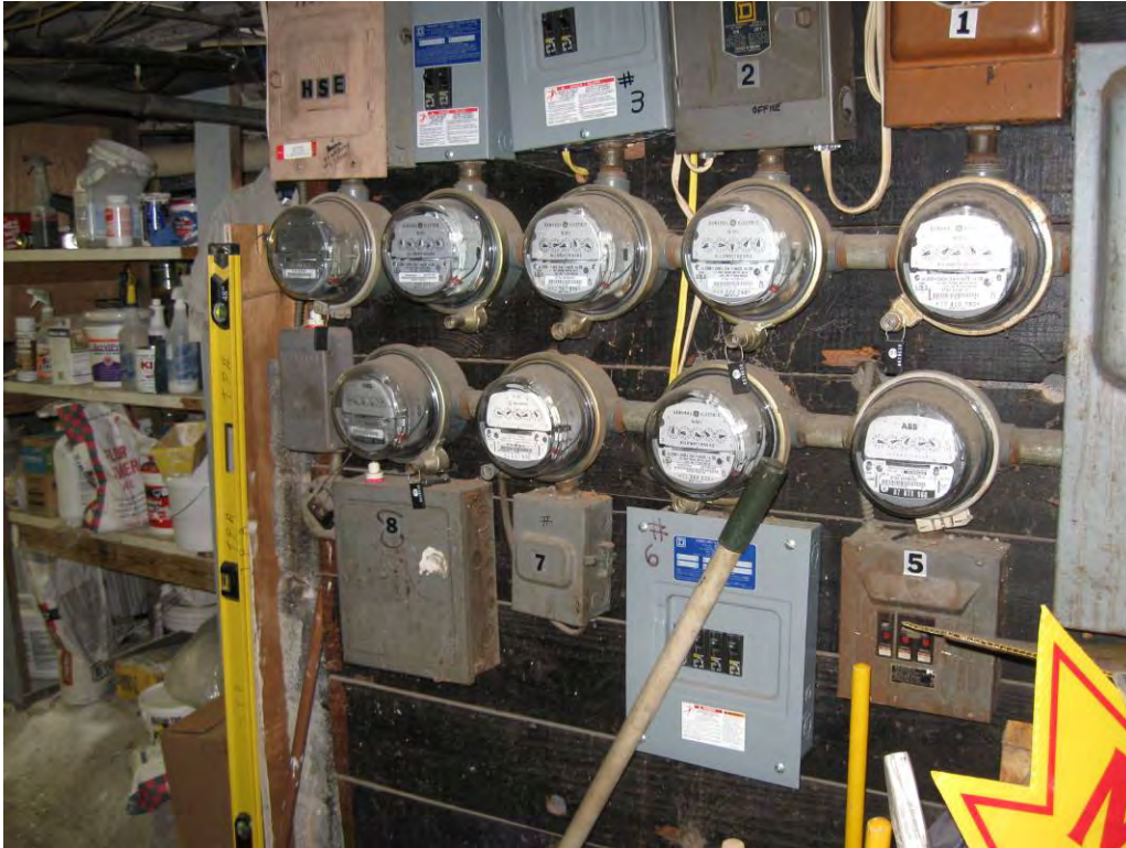
Additional electric service equipment for units that have a common heating system located in basement
