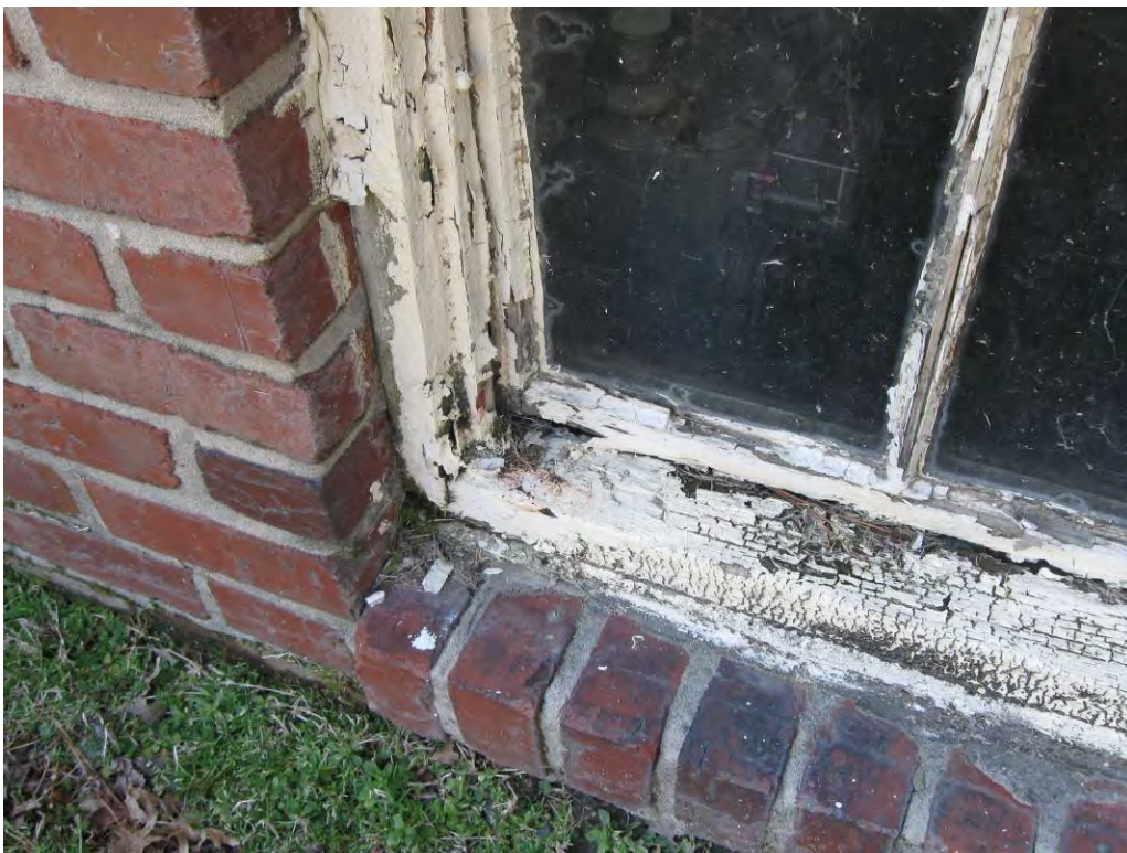
Basement windows require repair or replacement on many buildings (Bldg.25)
