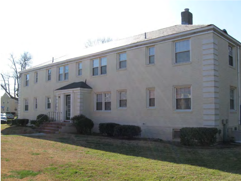
Building exterior, some buildings have a painted brick veneer
