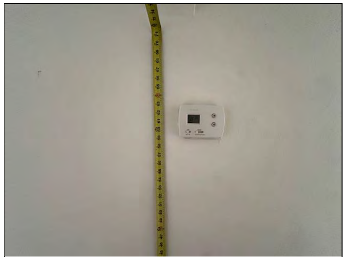
66. Thermostat mounted at 62" at center in apartment
