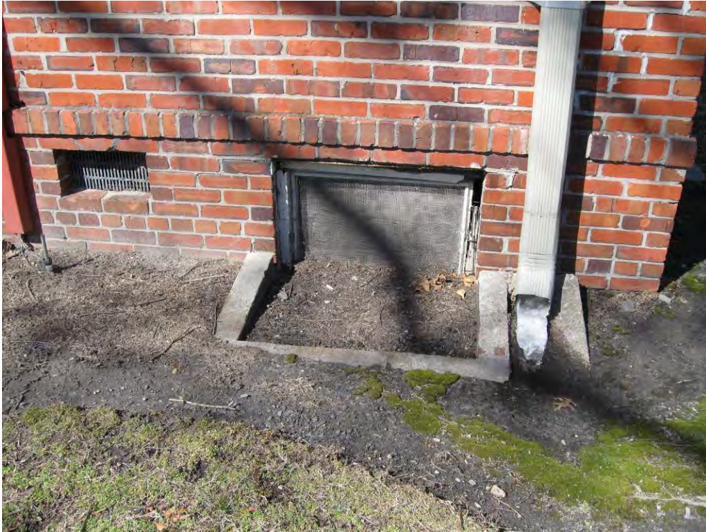
Basement windows require repair or replacement on many buildings (Bldg.32)
