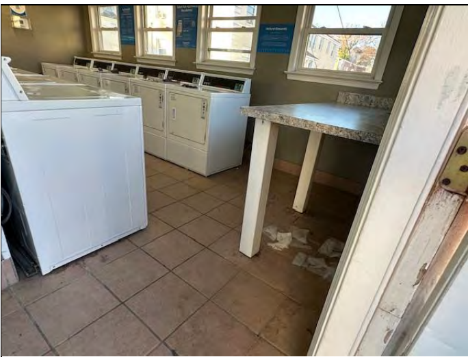
65. Laundry room walkway width at less than 32", and lack of access at folding table
