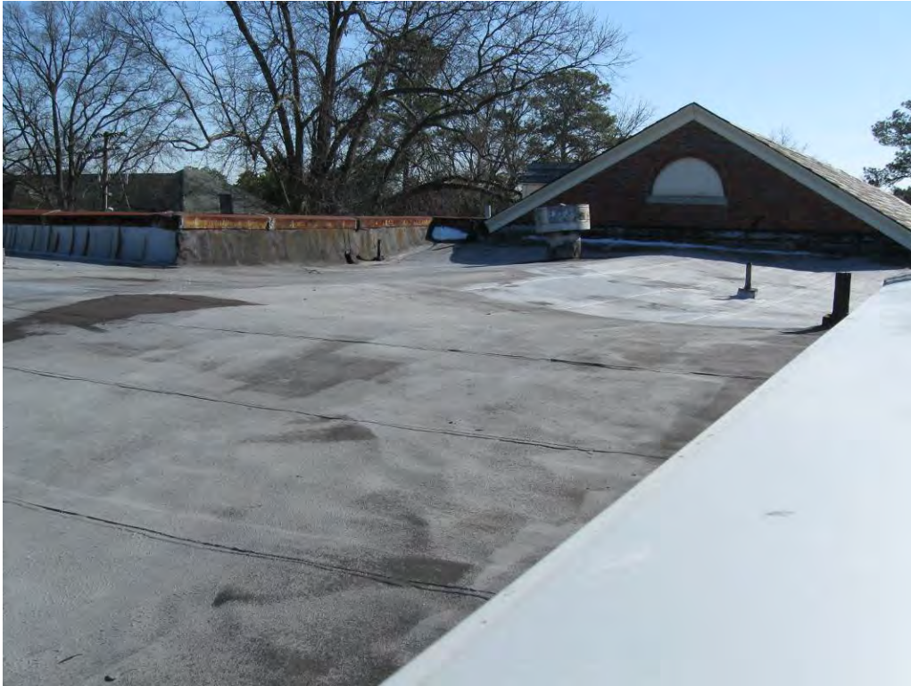
Flat rolled asphaltic roof covering on some buildings
