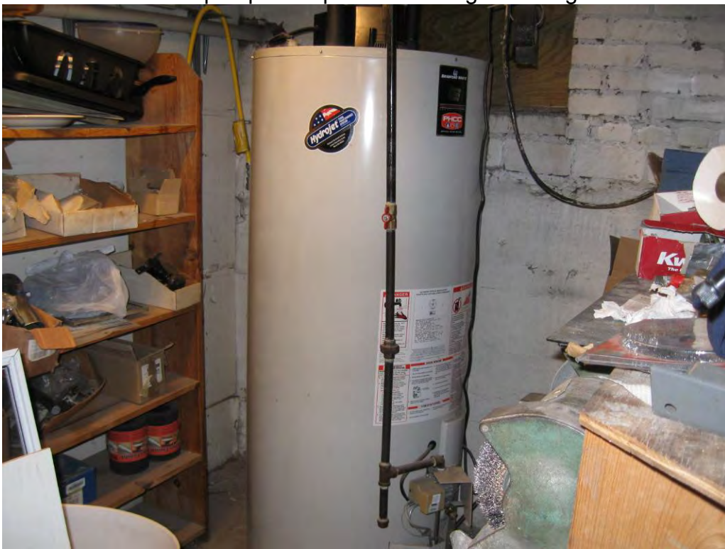
Common gas fired water heaters serve most buildings, galvanized water supply piping present
