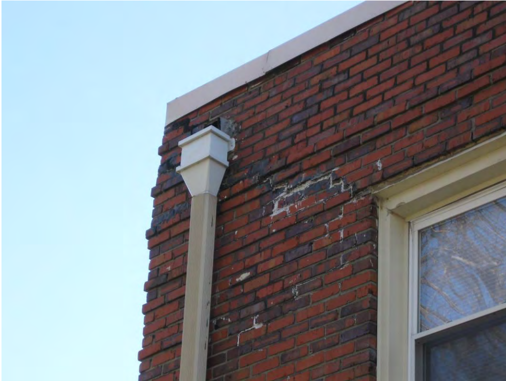
Brick veneer tuck pointing maintenance required on some buildings (Bldg. 27)
