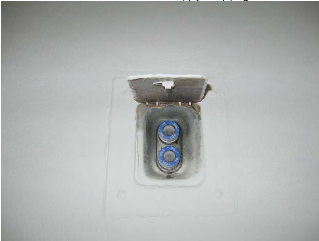
Fuse box present in units that have common heating system
