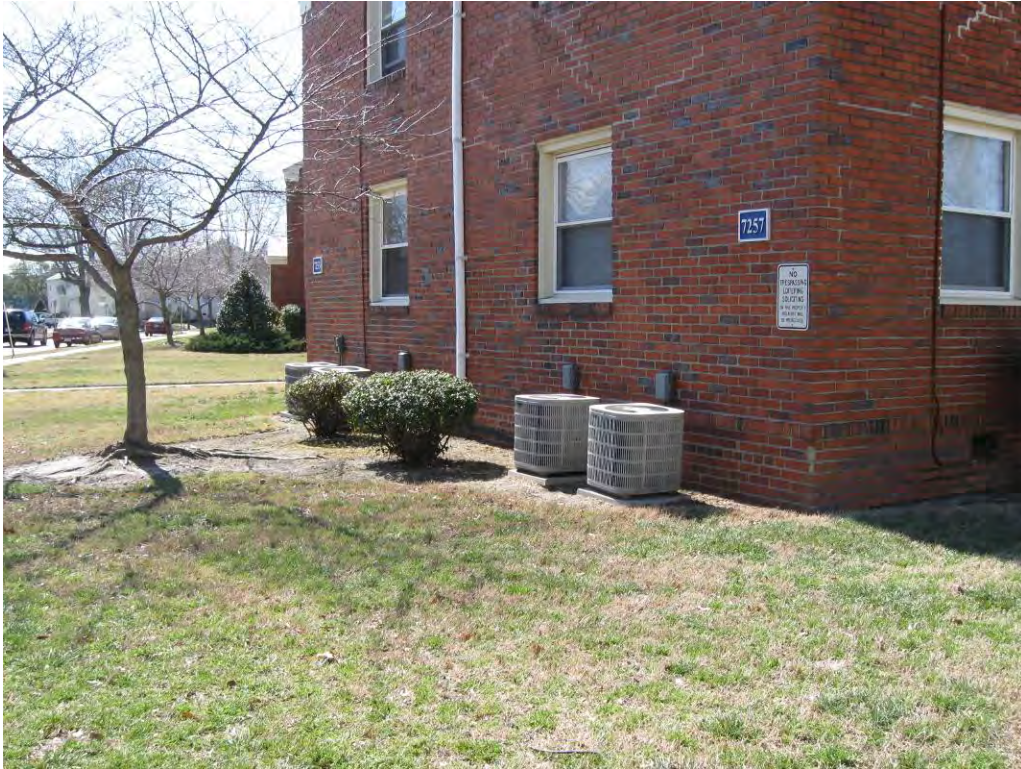
Some buildings have individual split system heat pumps that provide heating & cooling
