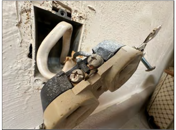
32. Copper electrical wiring observed in dwelling unit 2-22
