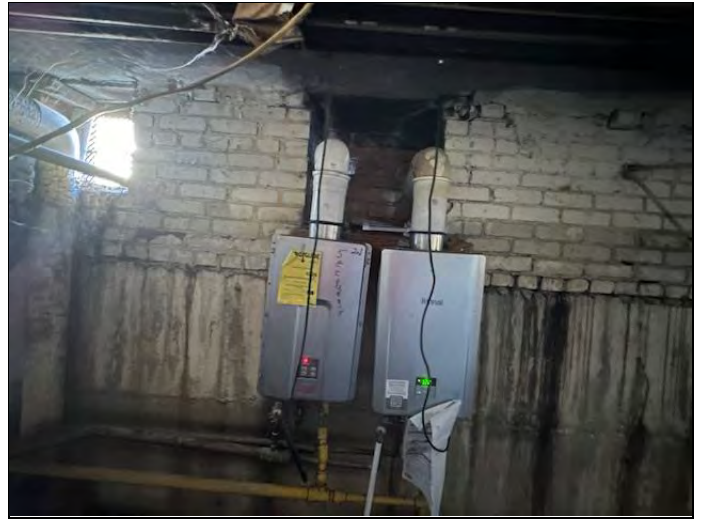
20. Gas-fired tank-less water heaters
