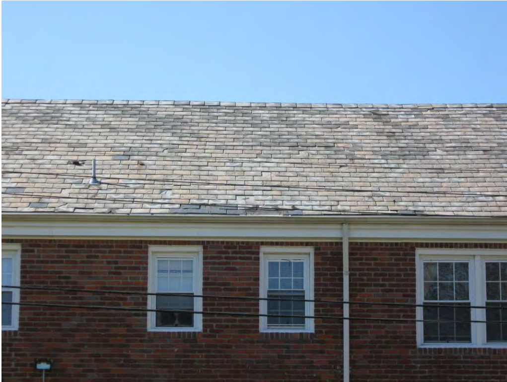
Slate roof shingles on most buildings
