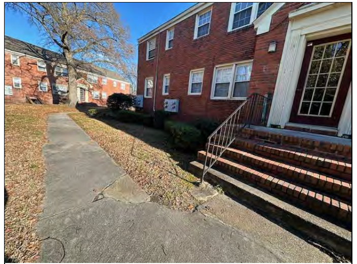
52. Representative damaged concrete sidewalk/trip hazard (near Bldg. 29)
