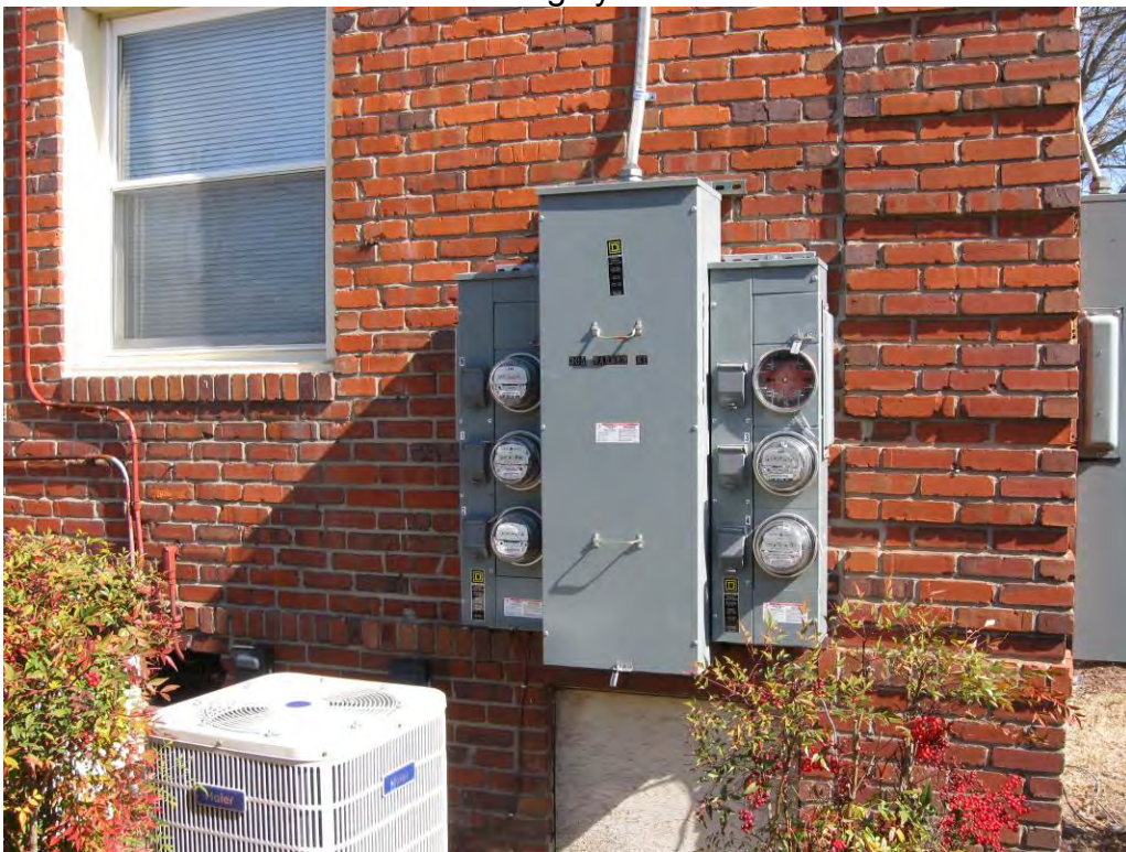
Electrical wiring upgrades for buildings that have heat pump systems (100 amps)
