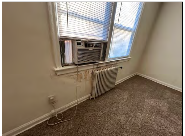
24. HVAC PTAC through the window unit
