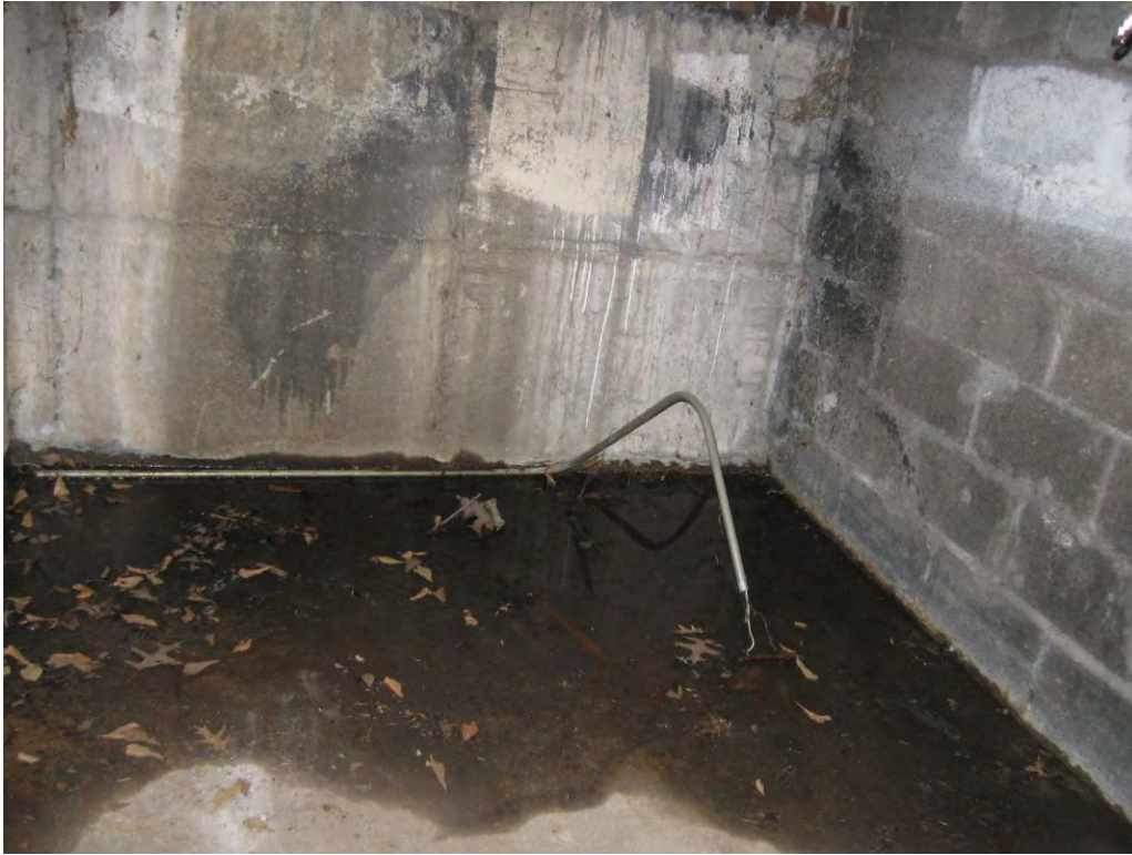
Evidence of water intrusion observed in some basements (Bldg. 32), no evidence of mold growth observed
