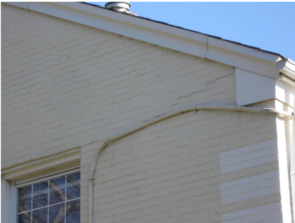
Brick veneer cracking, monitor and repair as required (Bldg. 28)
