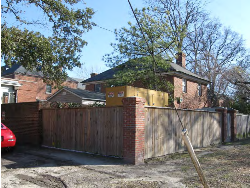
Self contained diesel fuel emergency generator located on eastern adjoining property
