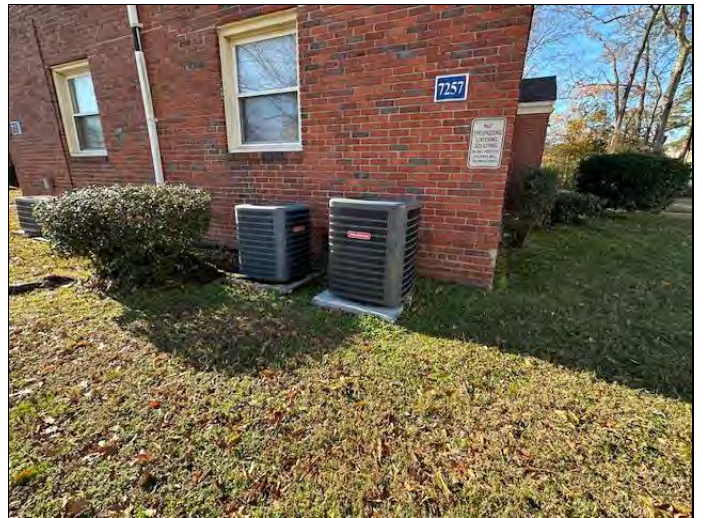
22. HVAC pad-mounted condensing units
