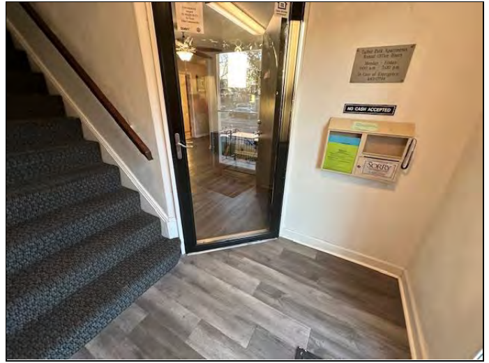
62. Leasing office entry door; note lack of 18" of clearance on pull side due to stairs
