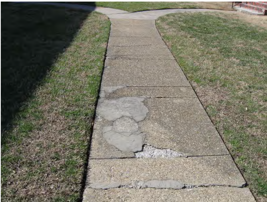
Concrete flatwork repair required in several locations (Bldg. 20)
