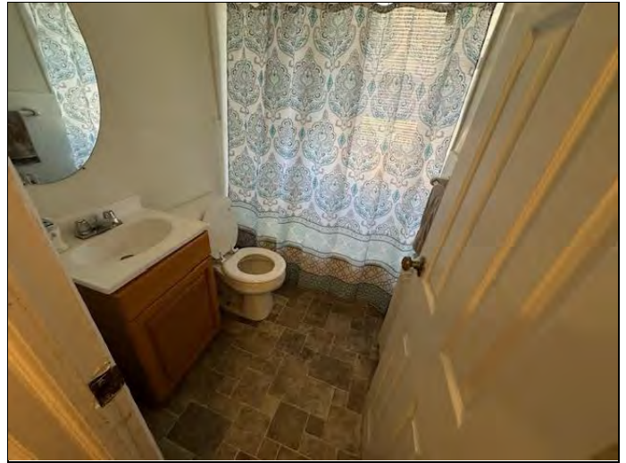
38. Leasing office/model unit bathroom; note lack of accessible features
