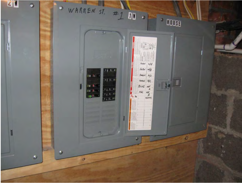
Circuit breaker panels located in basement for buildings that have heat pumps
