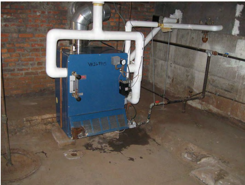
Some newer common gas fired boilers present
