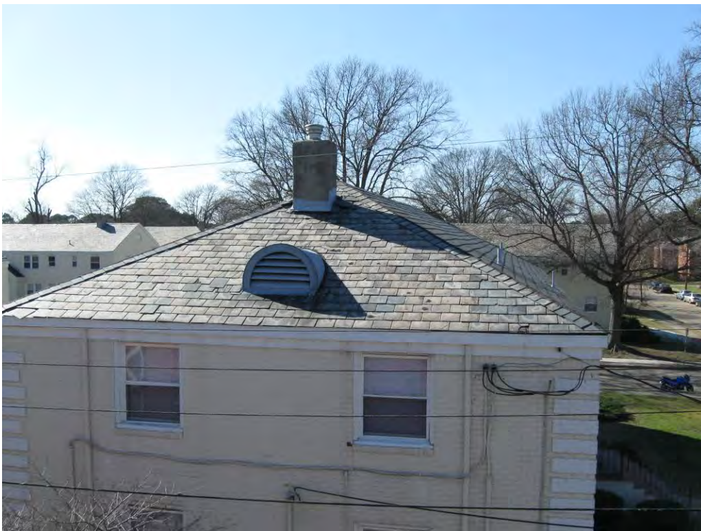
Slate roof shingles on most buildings
