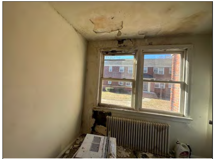
58. Damaged interior finishes and rotted window framing due to façade cracking (Bldg. 25, unit 6)
